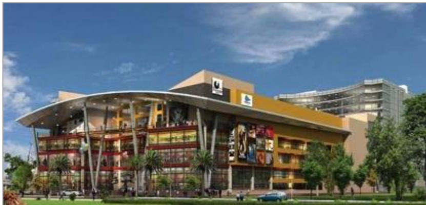
Forum Mall, 12,00,000 sq. ft. space that comprises of Shopping Mall, Office Spaces & Hotel in Chennai
